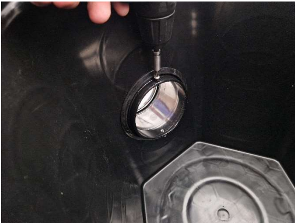
Install the inlet connection with a socket - secure against slipping out with INOX screws and rotate by 90°.
