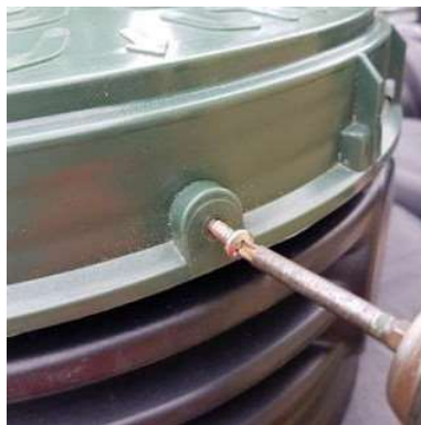
Place the screw in the hole. Tighten the screw
