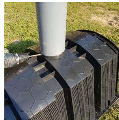
11. Install the vent
