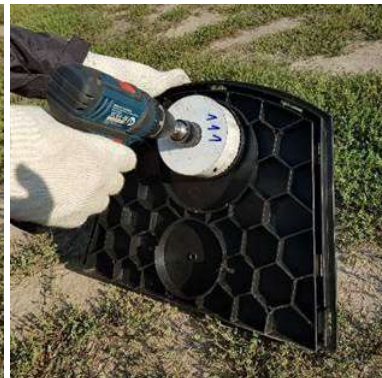
3. Drill a hole
