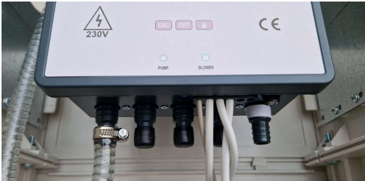
Figure 15: Keypad and LEDs indicating the operating states of individual controller outputs
