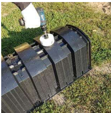
10. Drill a hole on the back
