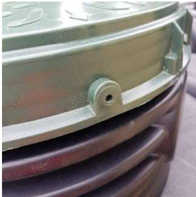
Screw on the cover. Locate the Safety hole.
