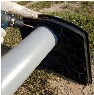
5. Secure with a screw
