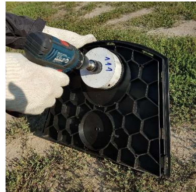
3. Drill a hole
