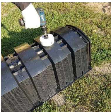
10. Drill a hole on the ridge
