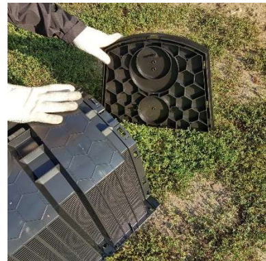
9. Plug the closing end plate
