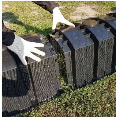
8. Connect the tunnels
