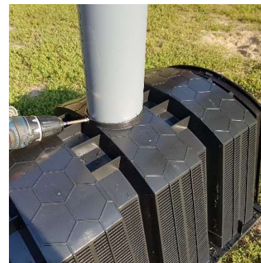
11. Install a stack
