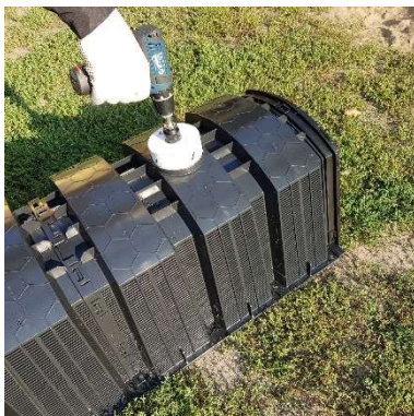
10. Drill a hole on the ridge
